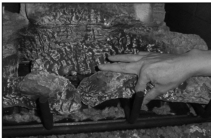
Figure 14.3 Placement of Rock Wool
